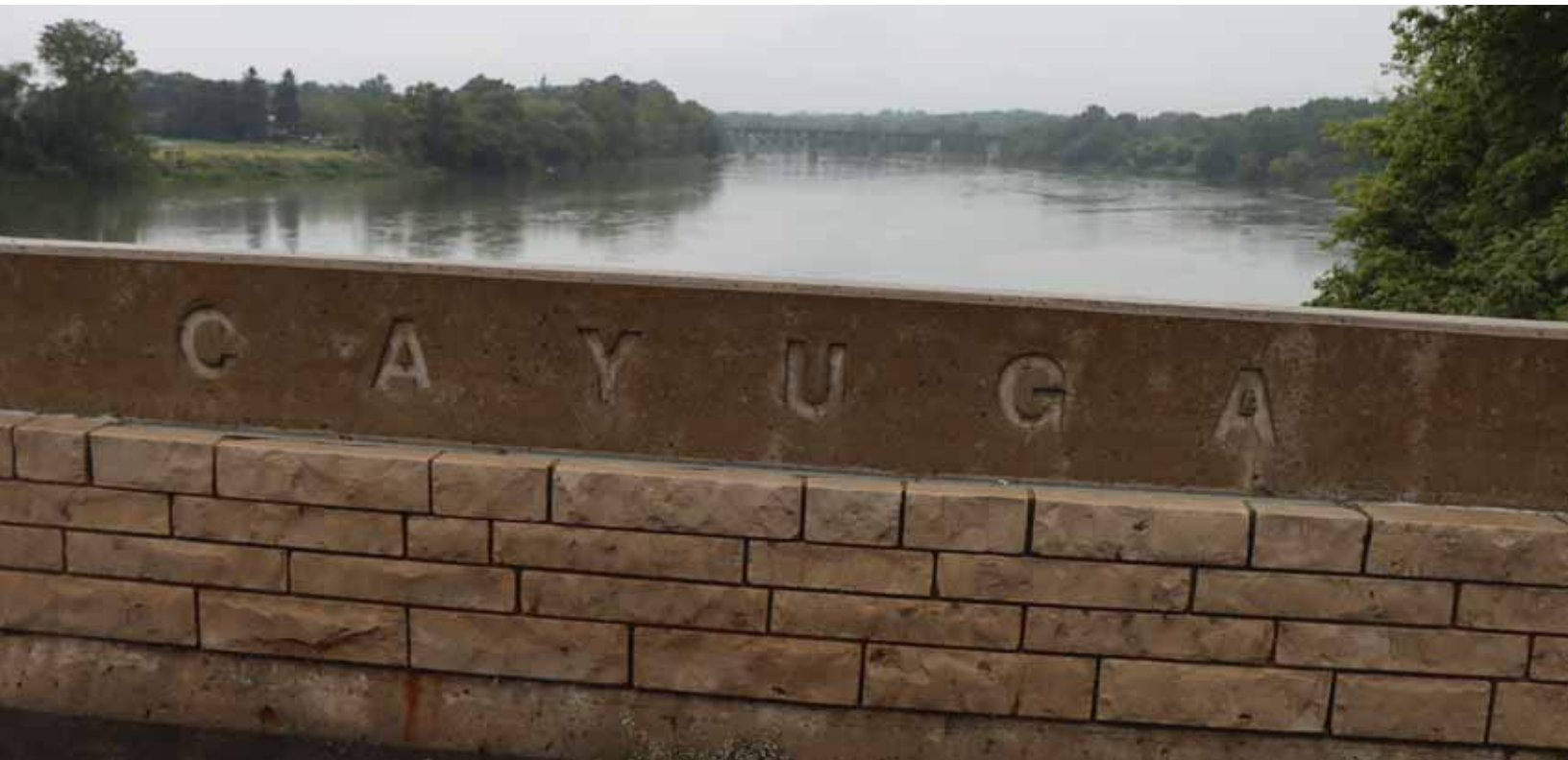
CAYUGA BRIDGE, CAYUGA, ONTARIO
